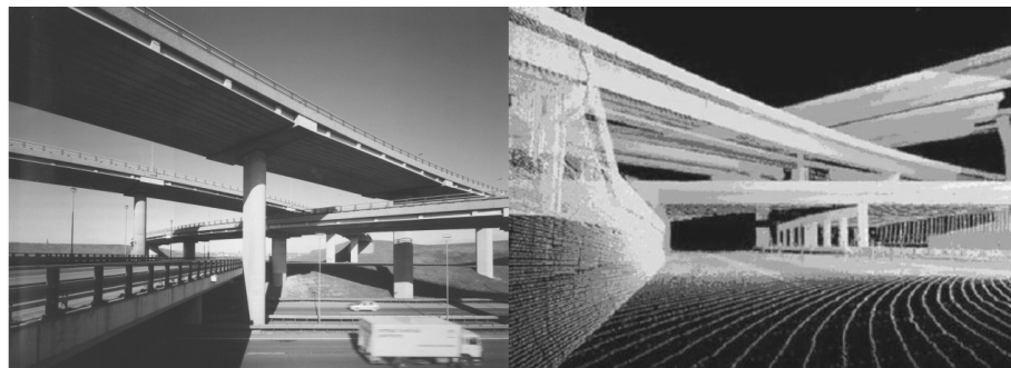
Fig. 2. Terrestrial laser scanning provides insight in complex objects
